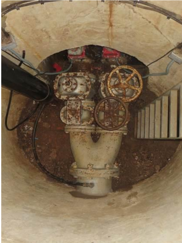
Photograph showing arrangement of valves. Remotely controlled butterfly control valves are those furthest downstream (top of photo)
