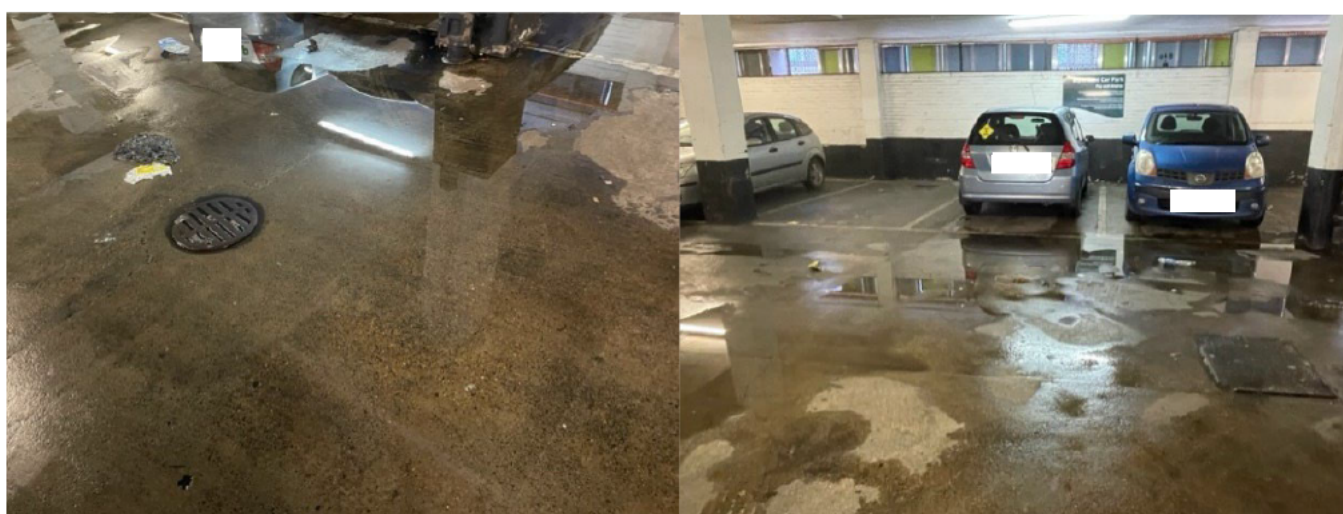
Floor Drains – Jetting out
